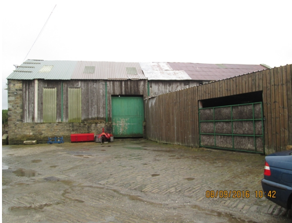
South elevation of Barn
