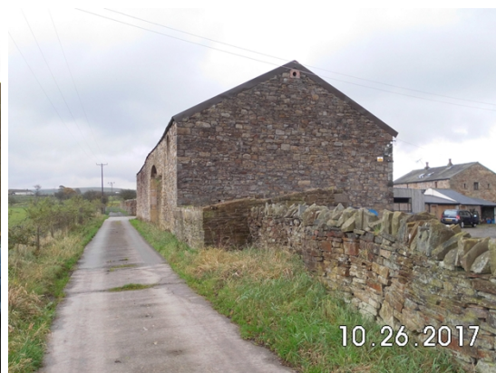
View of west gable and public footpath (along track)
